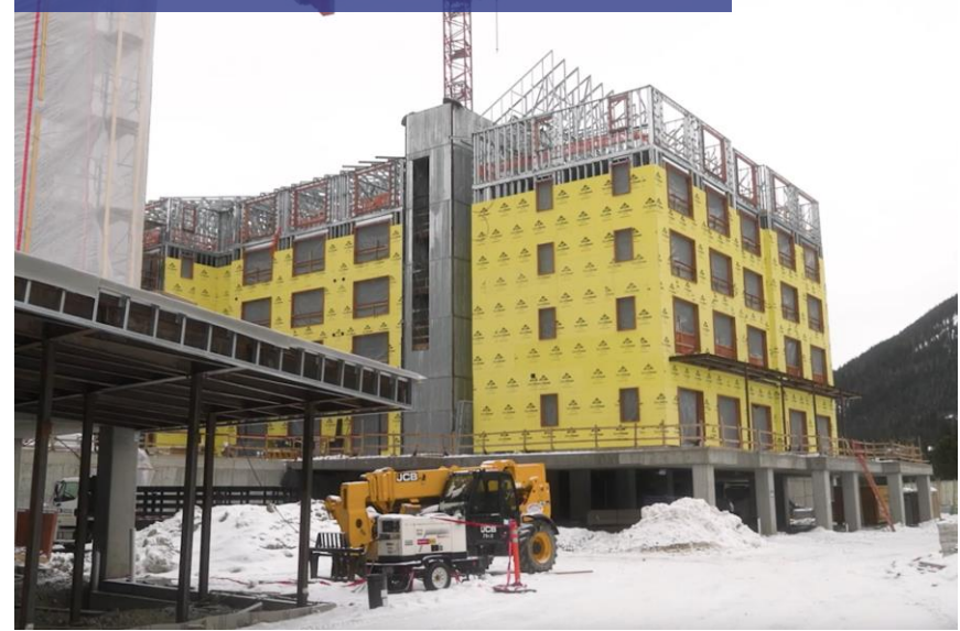
January 2024 Hotel Construction
