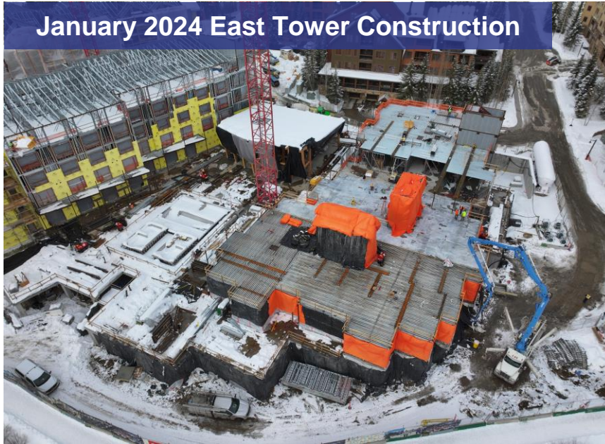
January 2024 Vertical Construction Progress
