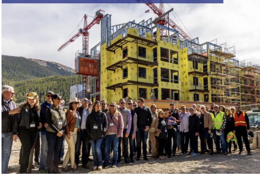
October 2023 West Tower Topping Out
